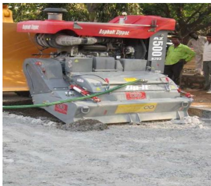
Fig. 4 Dry Mixing of RBI Grade 81, Watering and Wet Mixing Process
