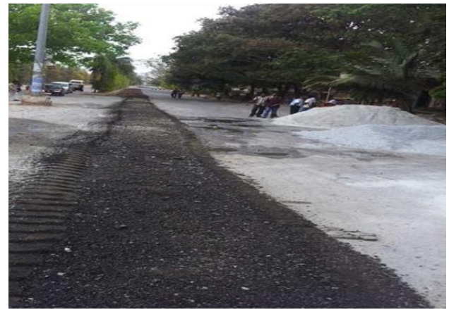
Fig. 2 Scarification process and scarified layer
