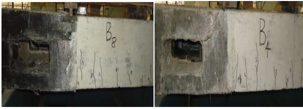
CFRP wrapping around and inside the opening
