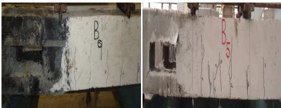
CFRP wrapping around the opening by double layer
