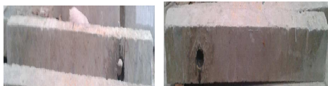
CFRP wrapping inside the opening
