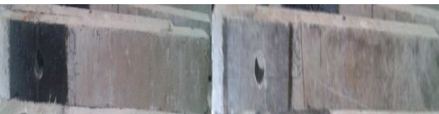
CFRP wrapping around the opening
