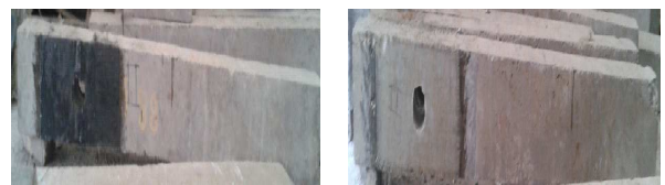
CFRP wrapping around the opening by double layer
