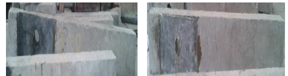
CFRP wrapping around and inside the opening
