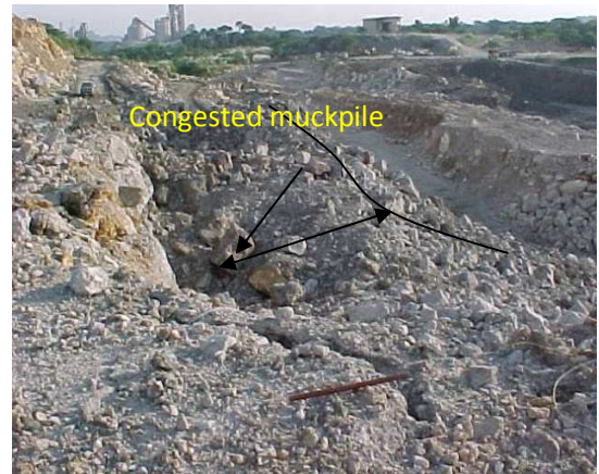
Fig.13: Excessive congestion of the blasted muck along the back rows (Diagonal firing)
