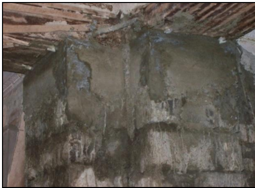
Fig -10: Grouting nipples at the top to fill voids
