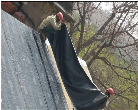
Fig -14: Laying of Multiplas sheet for waterproofing
