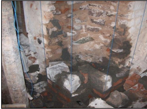
Fig -9: Reconstruction of partially collapsed column
