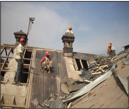
Fig -13: Dismantling of deteriorated roof members
