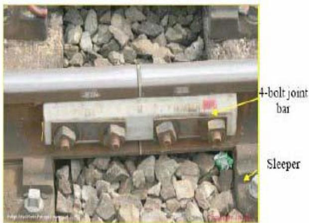
**Fig.1** A typical 4 bolt insulated rail joint
