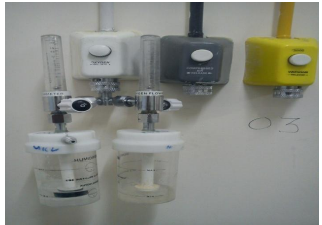
Fig 3.5 Shows Humidifier Circuit for Saturation
